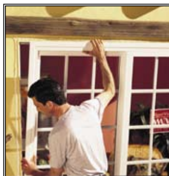
Step 2: Install new window INSIDE existing window frame.
