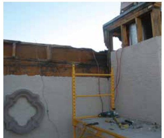
Above and below are examples of water infiltration damage.
