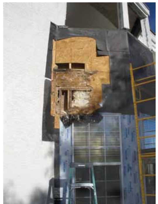
Above and below are examples of water infiltration damage.
